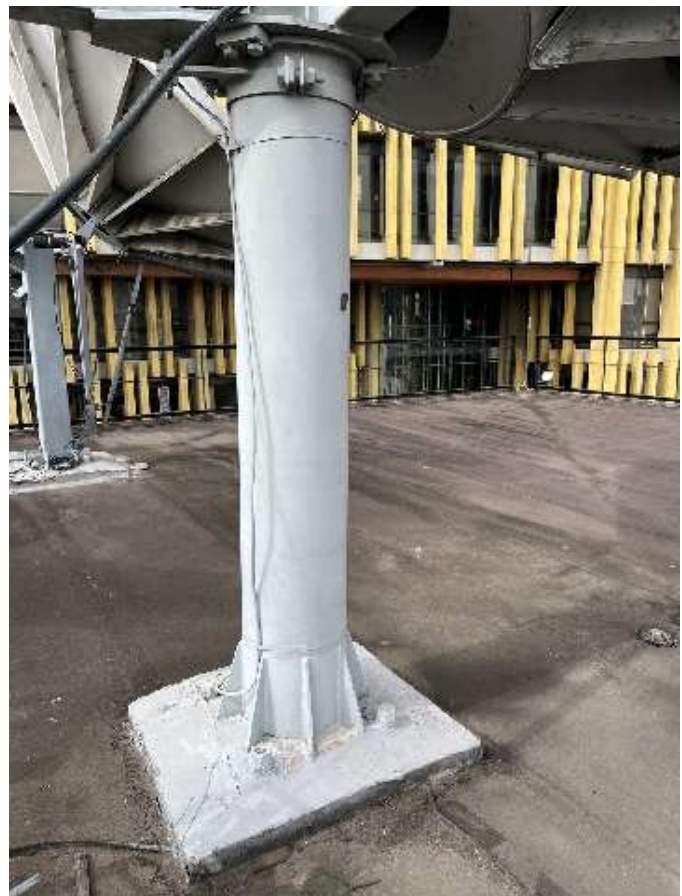
Antena principal Vertex 4.8 mts Cassegrain TX-RX Banda C circular
