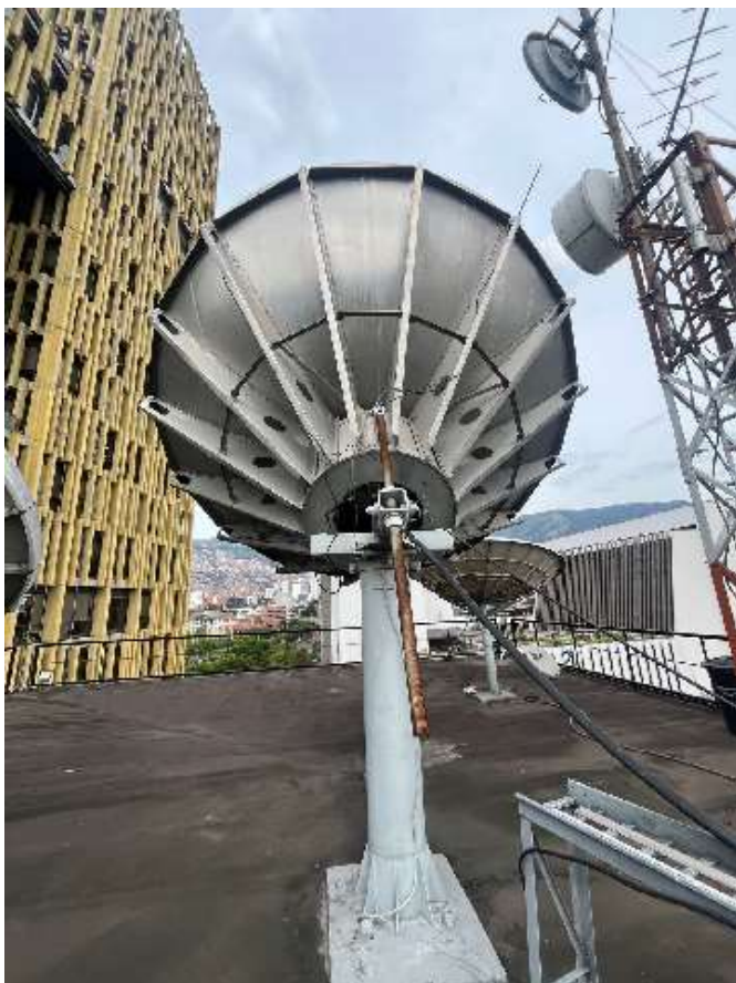
Antena principal Vertex 4.8 mts Cassegrain TX-RX Banda C circular
